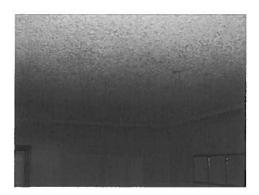
There is approximately 800 square feet of asbestos containing popcorn ceiling associated with the ceiling of this structure. This material runs throughout the house except for the bathroom, kitchen, and utility room.
